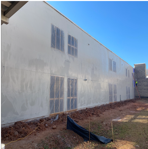
Completed exterior wall waterproofing in area 3
