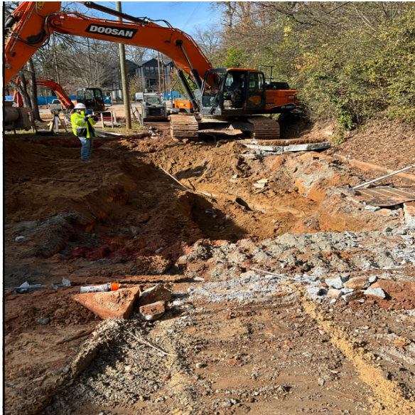
Continue prep for kitchen grease trap install
