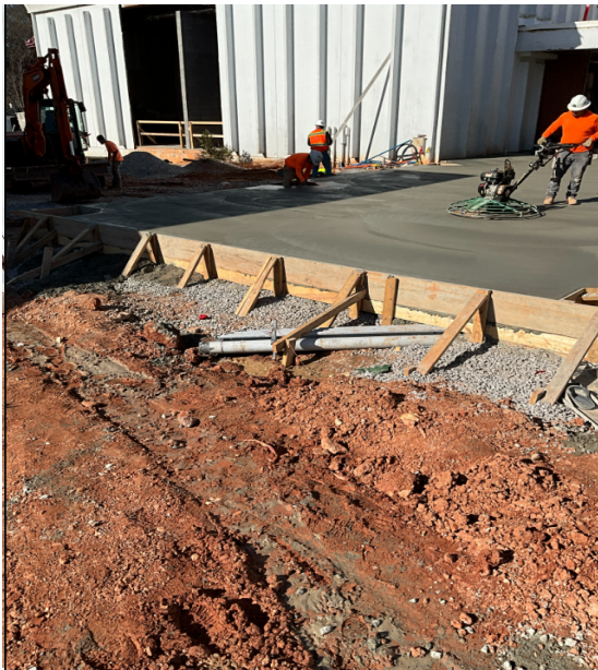
New security vestibule additions has poured and ready for steel
